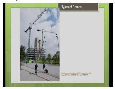
So, always for the erection of tower crane, you can see the mobile cranes are always standing nearby. It will help in the erection of the tower crane.
