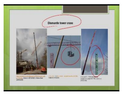
So, dismantling procedure of tower crane, say, if it is going to be climbing cage, it is going to be easy. If there is no climbing cage, we need the support of another mobile crane for the entire process. Say, first, you have to remove the trolley part you have to remove the trolley. So, after removing the trolley, you remove the counterweights. You remove the counterweights then you remove the jib. So, then you remove the counter jibs.
