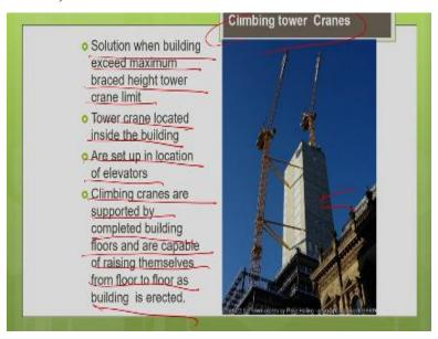
Say, for example, you need a tower crane for a structure which is greater than 300 meters. So, in that case, what is the option available? There are certain special cranes called as climbing tower cranes which can grow along with the structure. These grains are generally shorter but it will grow along with the structure. So, basically, what this climbing tower grains will do is; it will take the support from the actual structure which you are going to construct.
